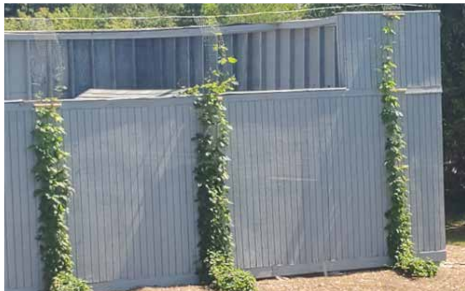
On the grounds of the Cook County Farm Bureau, a few new plants are being established. With the need to provide green cover to the chiller/garbage structure following the removal of overgrown shrubs, the Building Committee thought that they might see if hops would fill the need. Once established, the plants have grown quickly.
